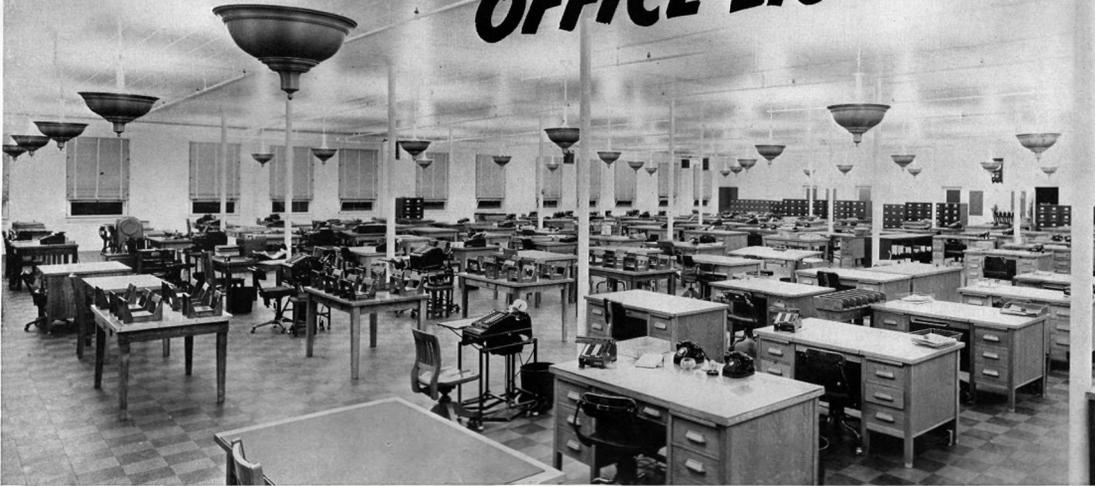
● The newest thing in office lighting is this combination of mercury and incandescent lamps in the general office of the Cannon Mills at Kannapolis, N. C. Each of the totally indirect luminaires contains one 400-watt mercury lamp and four 200-watt Mazda lamps. Illumination of about 30 footcandles is provided.
